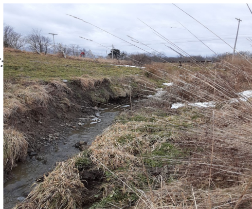
Eroded stream bank
